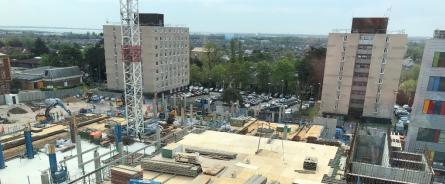
**Construction update:** All preparatory works have taken place and groundworks and foundation are now 75% completed. Over 3,000 tonnes of concrete has been recycled and used to build the groundworks and foundations of the new building.
